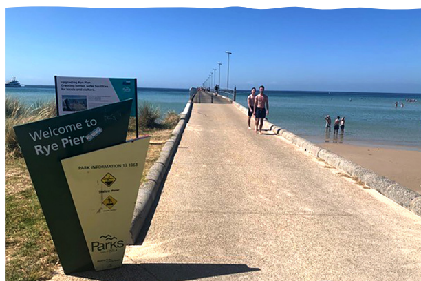
Image: Rye Pier stage one works
