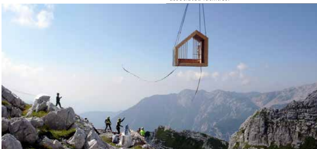
Prefabricated shelter transported to site.
