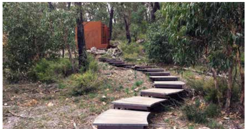
Design integrated WC units, Bugiga Camp Site, Grampians
