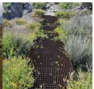
Use of open steel grates to enable plant growth underneath.
