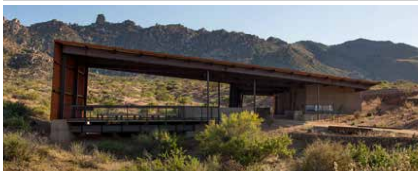
Tom's Thumb Trailhead, McDowell Sonoran Preserve. Arizona, USA. Fucello Architects Photo credit: Bill Timmerman
