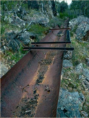
Stawell Water Supply Fluming. Courtesy of DSE.
