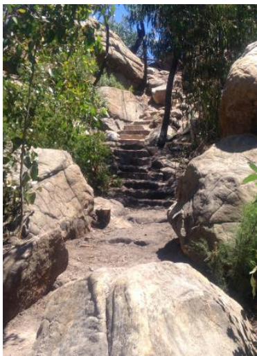
New rock work along Mt Difficult
