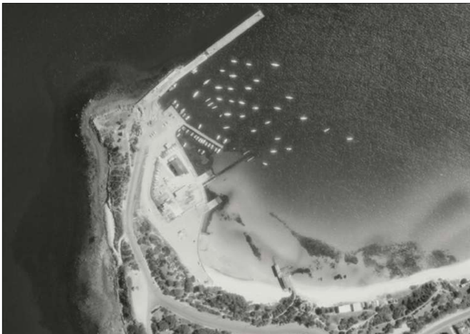
Figure 21 Aerial image, 1975. The Yacht Club clubhouse had been constructed by this time. Source: www.landata.vic.gov.au
