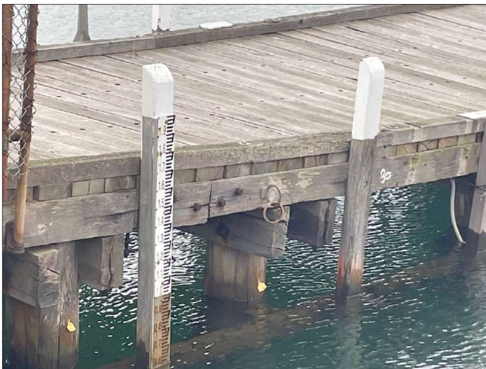
Figure 33 Fisherman's Jetty showing typical construction method.
