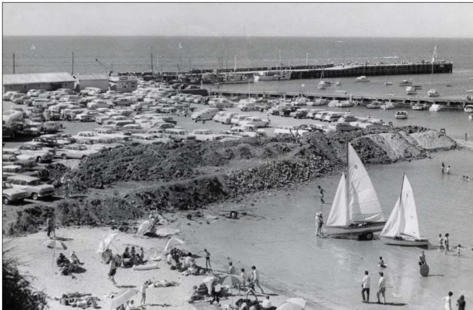
Figure 19 Land reclamation underway south-west of Fisherman's Jetty, 1960s Source: Mornington & District Historical Society.
