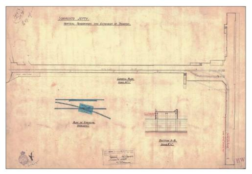
Figure 131905 drawing for extension of the tramway along the pier head.Source: Nepean Historical Society
