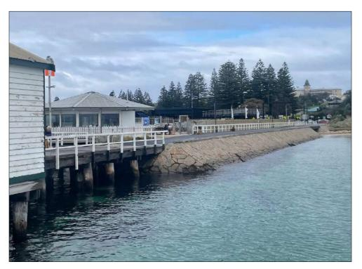
Figure 34 View from the pier looking towards the foreshore. Note the stone mole replacing much of the original timber pier.
