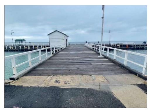
Figure 30 View of the pier where it transitions from the stone mole to the timber T-head.
