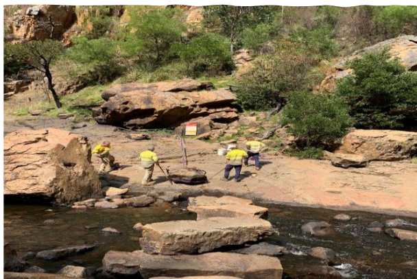
Photo 1 – Rock stepping stones to unsafe area being removed.
