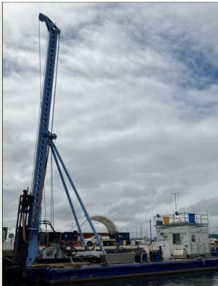
Figure 2: 18m pile driving barge utilised for works
