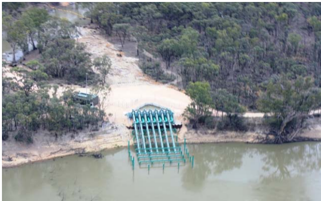
Messengers Pump Station
