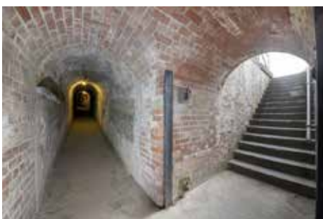
8. Tunnels – Fort Nepean Credit: John Gollings
