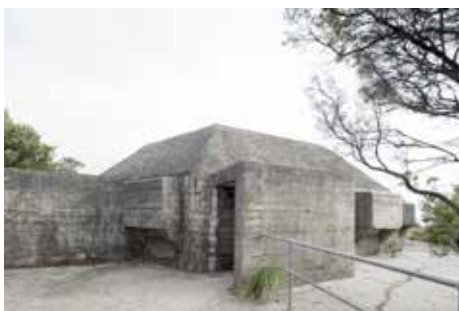
5. Gun Emplacement 6 – Entry Credit: John Gollings
